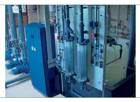
The CHLORINSITU® II range of electrolysis systems generates sodium hypochlorite with a concentration of 5 g/l. Our systems are especially suitable for applications where a robust and clearly understandable technology is required and where it is unproblematic if sodium chloride ends up in the water to be treated.
